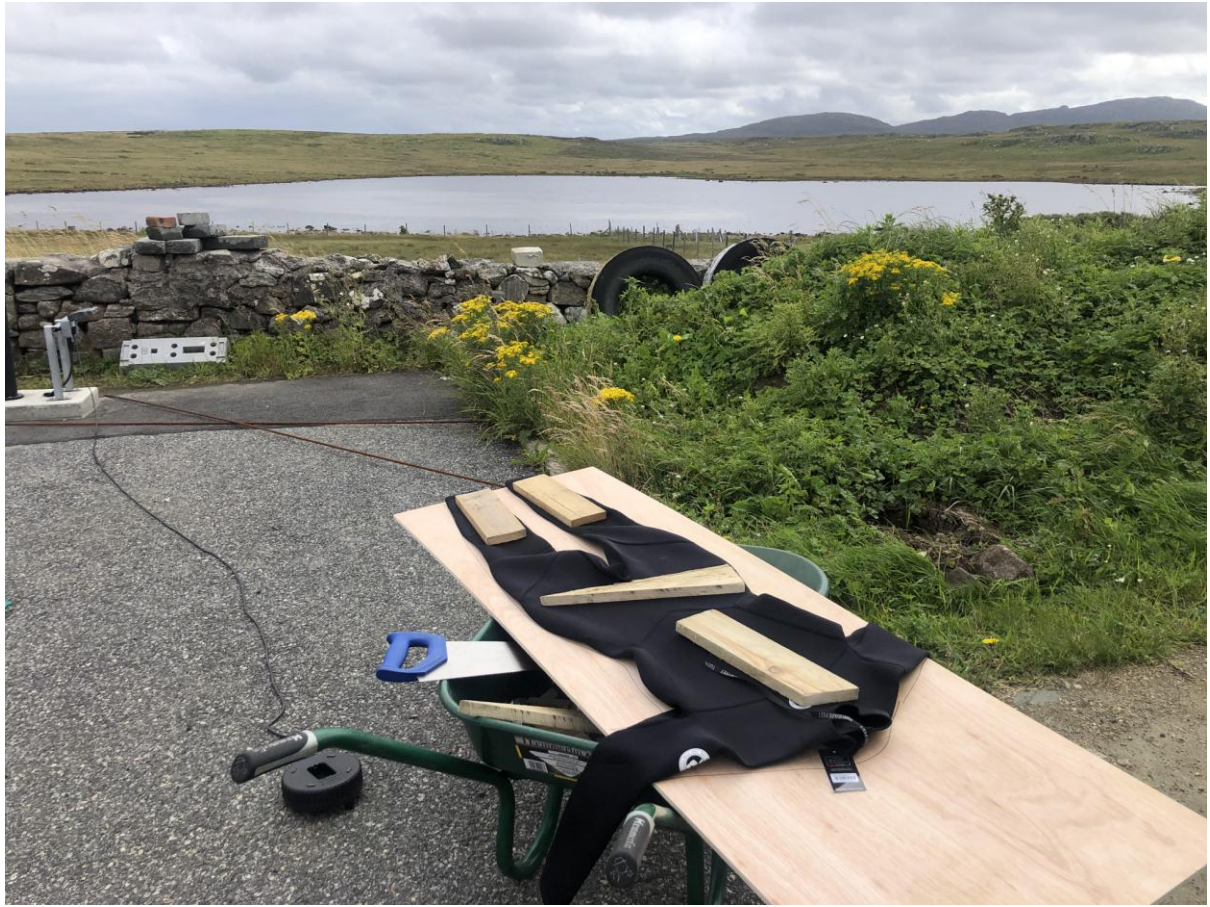
Making a wooden template for Raft1, Grinneabhat, Bragar.
